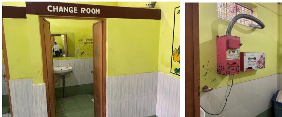
Changing room with incinerator and sanitary pad vending machine Chengail Shree Vidyaniketan High School, Uluberia
