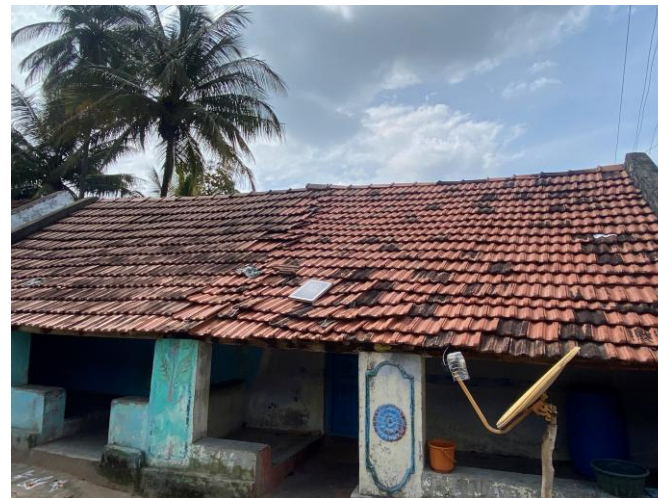
Solar panels installed in houses
