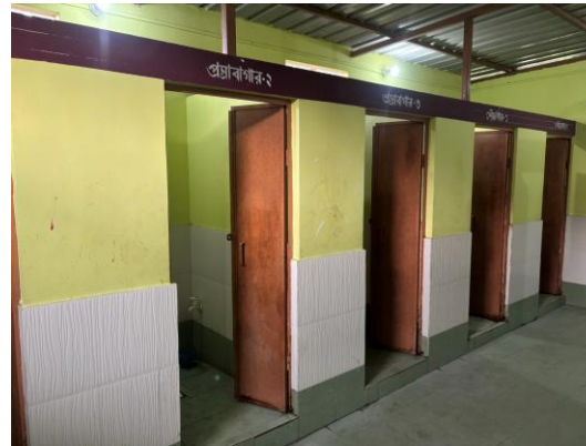
Newly constructed toilet block at Khaskhamar High Madrasah, Uluberia
