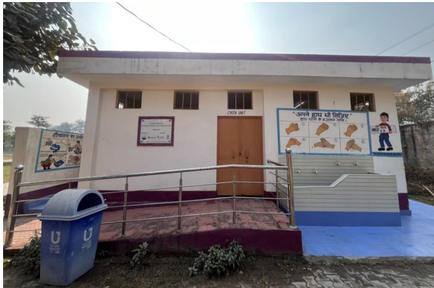
Newly constructed toilet block at Government School, Mirtzapur
