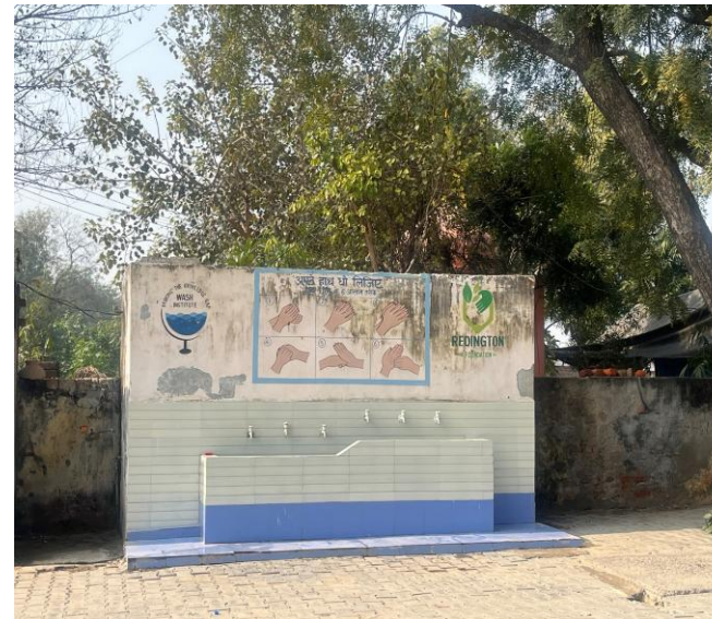
Drinking water stations at Government School, Kurali
