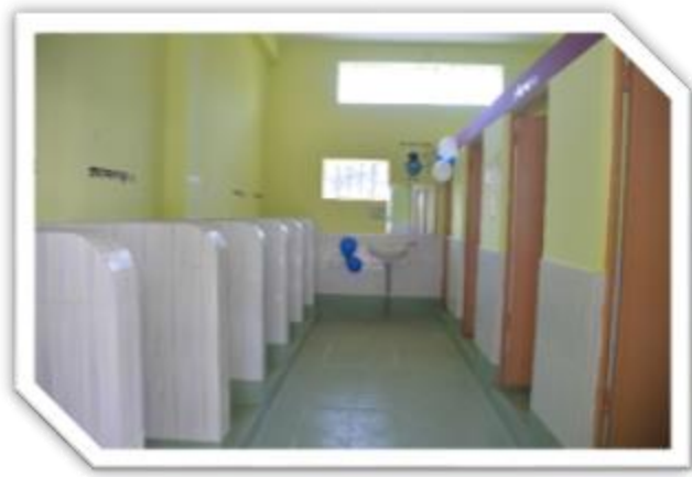
Toilets Constructed in Schools- West Bengal & Haryana
