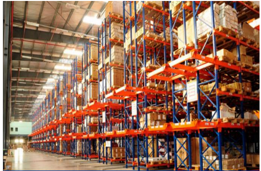
RACKING SYSTEM INSIDE ADC
