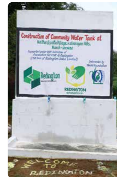
Through Constructing 4 rain water harvesting structures we established water storage tank with a capacity of storing - 52 Kilo Litres
