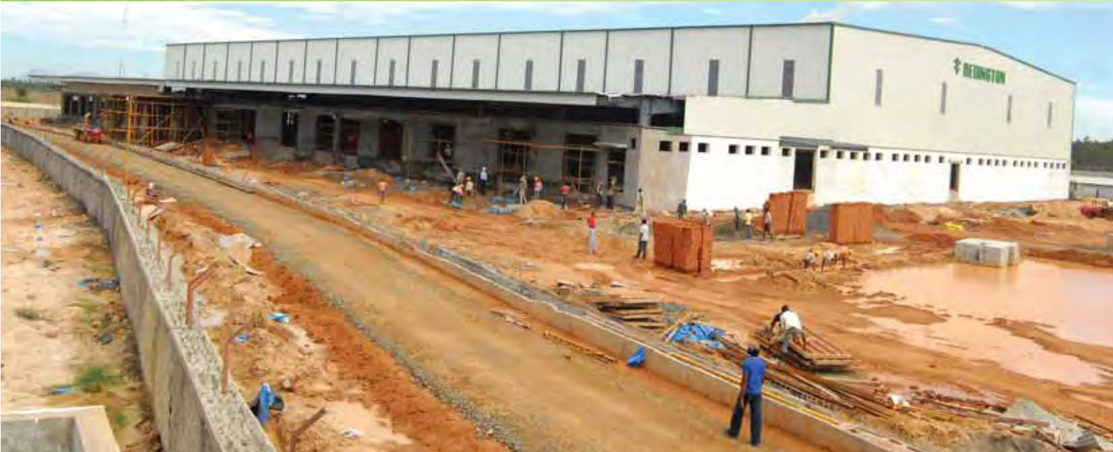
Automated Distribution Centre, at Chennai - Getting ready.
