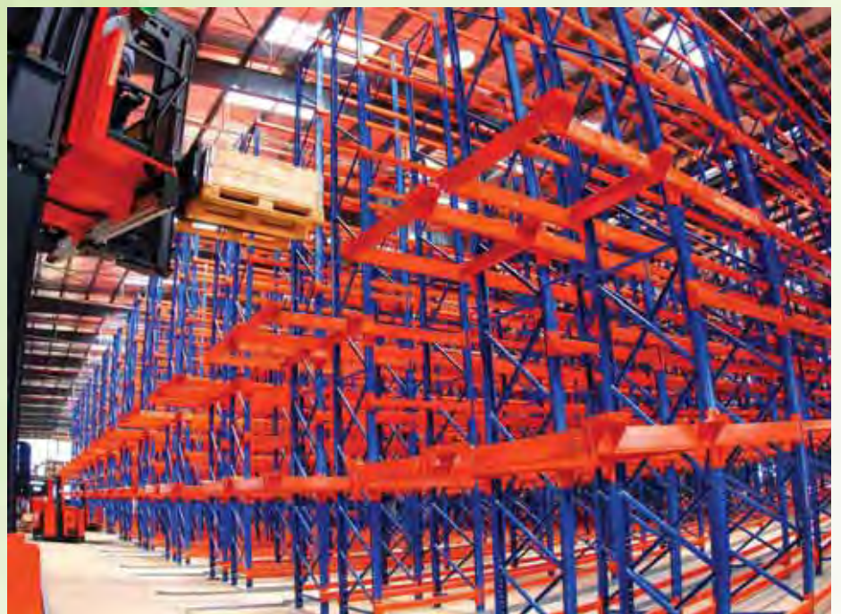
An inside view - VNA equipment and MHE under test.
