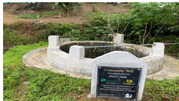
Well Restoration – Kalvarayan * Jawadhu Hills
